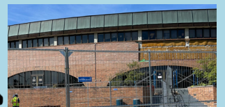
Reconstruction of the brick wall. PHOTO BY SATVIKA RAMANATHAN
